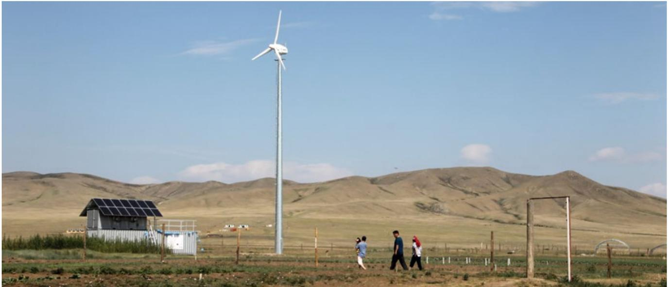
As part of the dena RES Programme, an off-grid hybrid system was installed at a research and training facility of the Mongolian University of Life Sciences. It combines a small wind turbine, a PV plant, an emergency back-up generator and a storage system.
